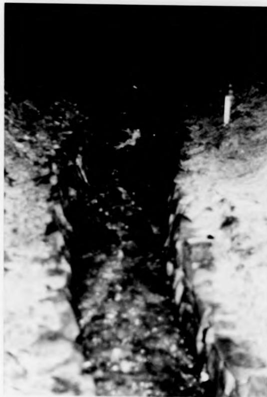
PLATE 2.3.1 (a) Coombs Brook catchment. Stone-pitched channels laid in the downstream reaches.
