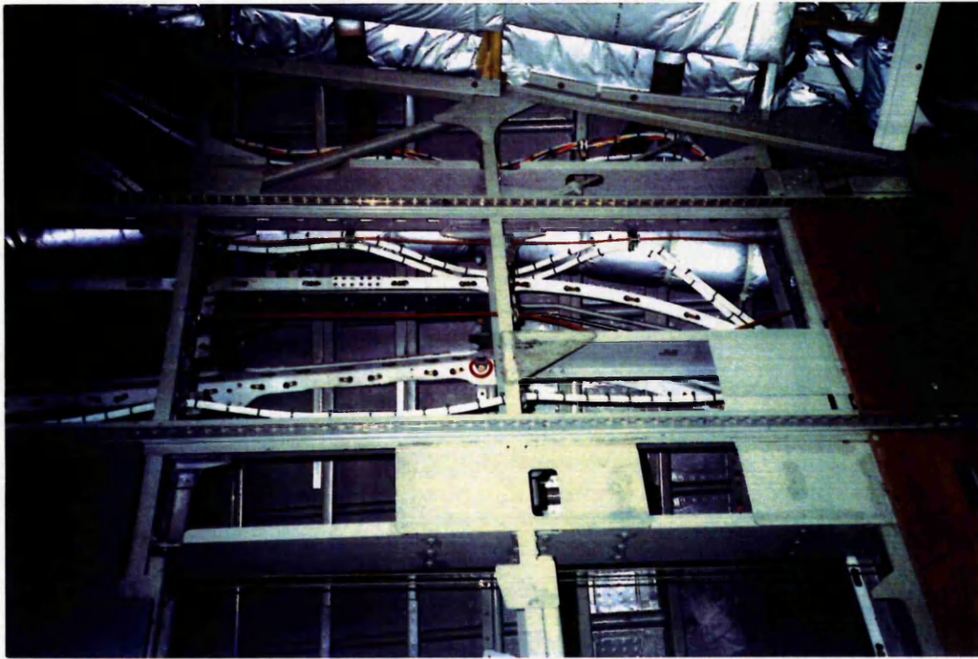
Plate A5.2 - 3R Modular Underfloor Support Structure
